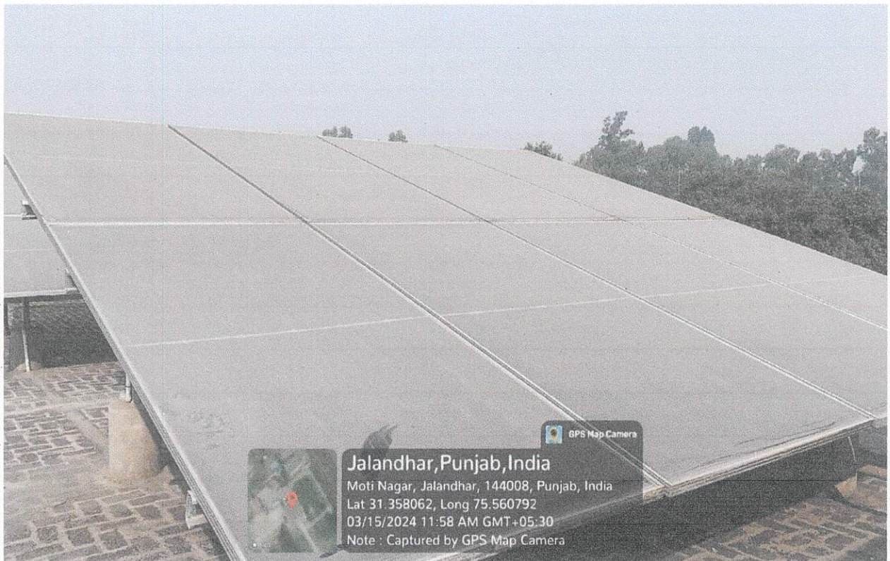
Solar Panel are installed on Rooftop
